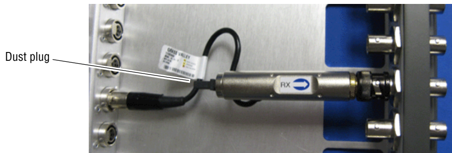
Figure 20. Installing MVMC Module
