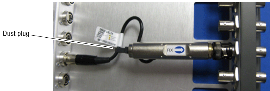
Figure 13. Installing MVMC Module
